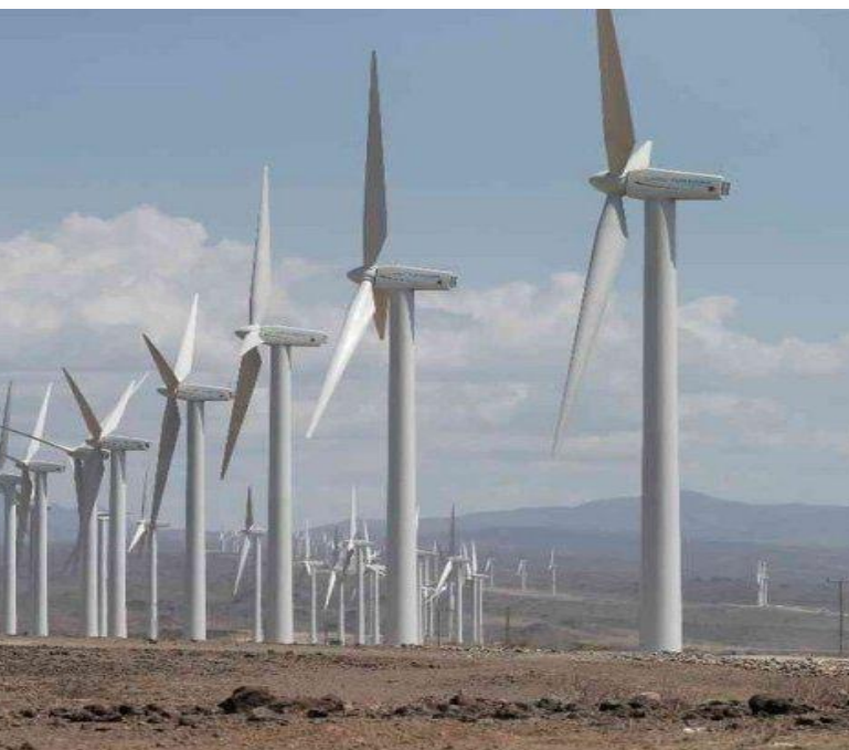
Figure 4: Image of completed Wind Turbines at Kipeto Wind Farm
